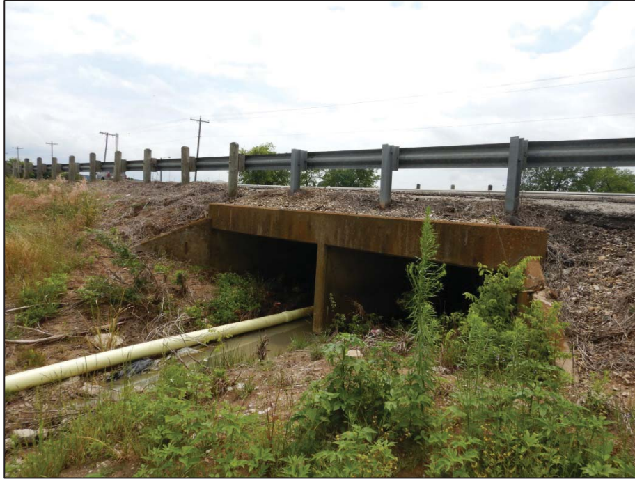
Photo 101: View looking west toward Crossing 16 – tributary to Cantrell Slough (US 377 northbound side).
