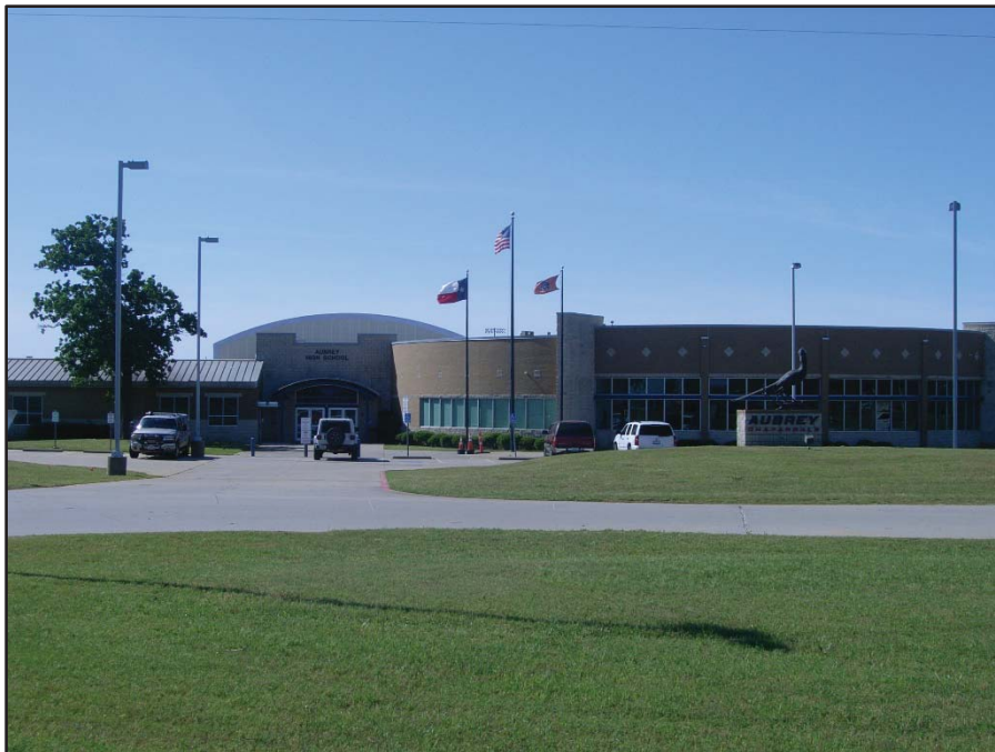
Photo 10: View looking south from Spring Hill Rd towards Aubrey High School (ID 54) at 510 Spring Hill Rd, Aubrey, TX 76227. Date of Photo: 4/29/20.
