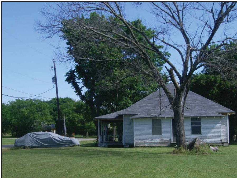
Photo 30: View looking north from E Walcott St in Pilot Point toward a home in disrepair. Date of Photo: 5/6/20
