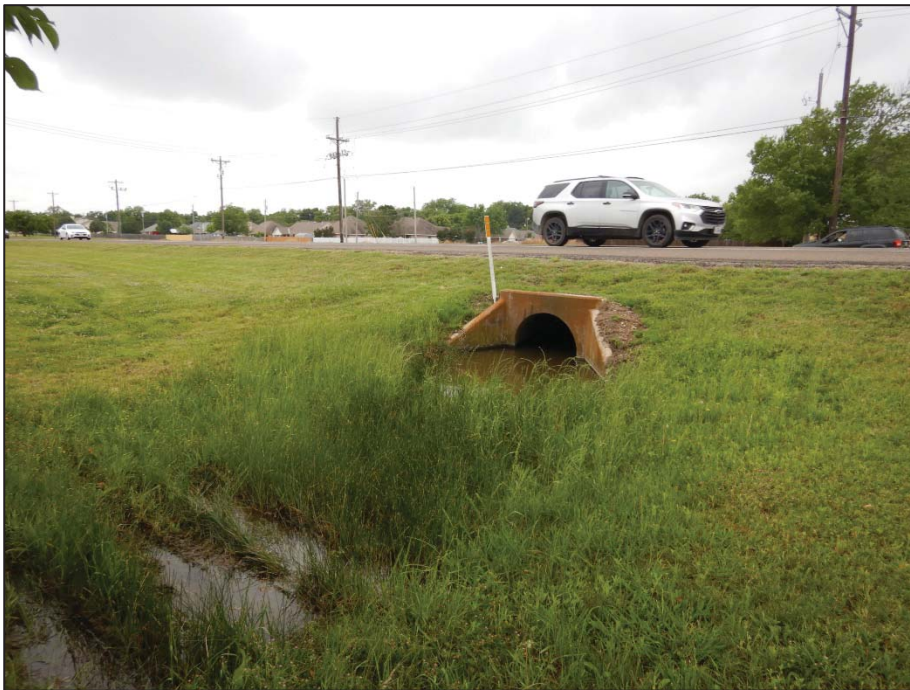
Photo 88: View looking west toward Crossing 12B – tributary to Pecan Creek (US 377 northbound side).
