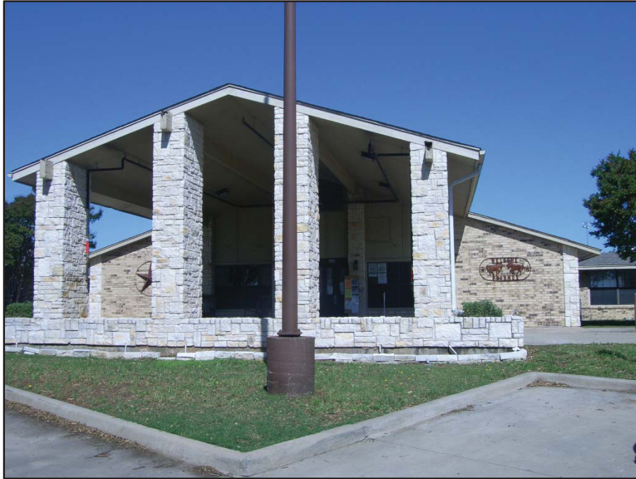
Photo 1: View looking northwest from a parking lot off Business 377 towards Countryside Nursing & Rehabilitation (ID 3) at 1700 N Washington St, Pilot Point, TX 76258. Date of Photo: 4/29/20.
