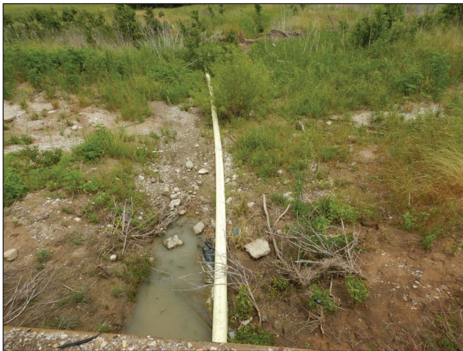
Photo 102: View looking east toward Crossing 16 – tributary to Cantrell Slough (US 377 northbound side).
