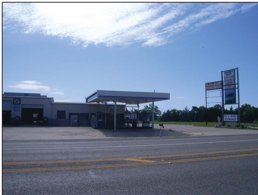
Photo 20: View looking southeast from US 377 toward Sunny Mart, a potential displacement (Disp. 2) at 1293 S US 377, Pilot Point, TX 76258. The site is a moderate environmental risk. Date of Photo: 5/6/20
