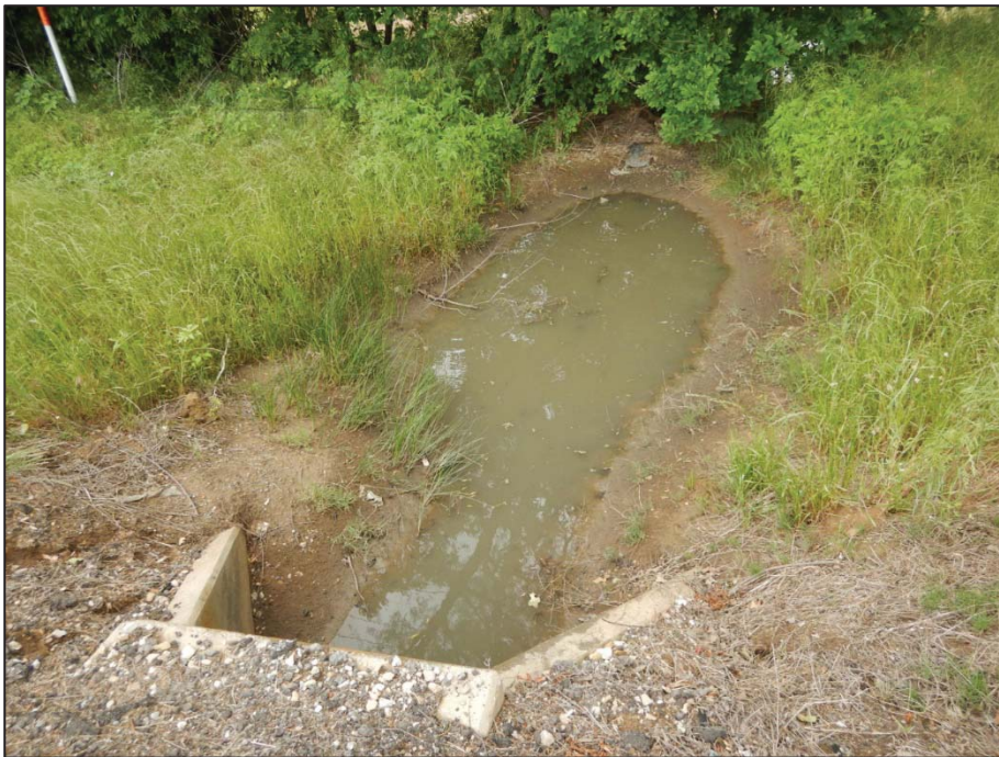
Photo 98: View looking east toward Crossing 15 – tributary to Cantrell Slough (US 377 northbound side).
