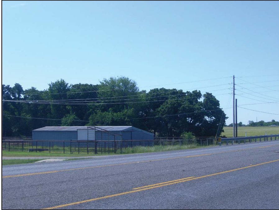
Photo 21: View looking southeast from US 377 toward a metal barn that is a potential displacement (Disp. 3) at 1311 S US 377, Pilot Point, TX 76258. Date of Photo: 5/6/20
