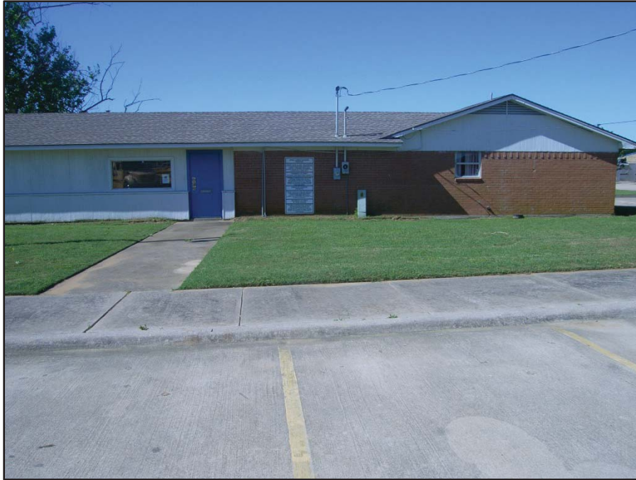
Photo 9: View looking southwest from a parking lot off US 377 towards the Aubrey ISD DAEP (ID 42) at 415 Tisdell Ln, Aubrey, TX 76227. Date of Photo: 4/29/20.
