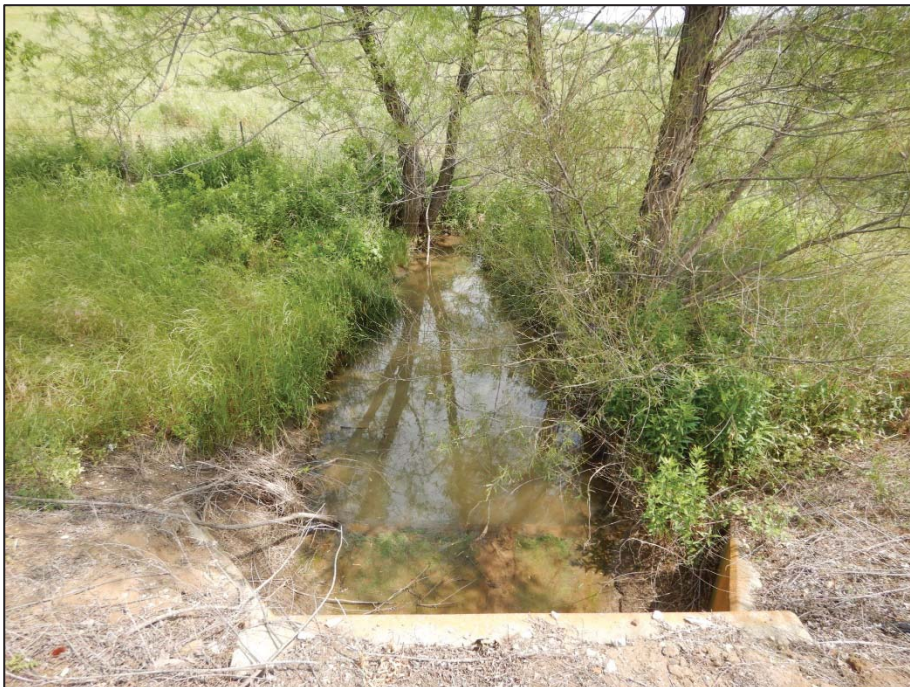
Photo 104: View looking southeast toward Crossing 17 – tributary to Cantrell Slough (US 377 northbound side).
