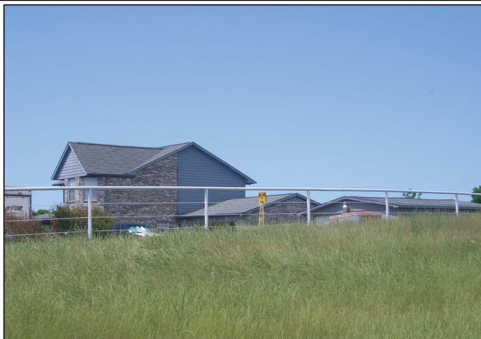
Photo 46: View looking southwest toward a natural gas pipeline marker along Fishtrap Road just west of US 377. Date of Photo: 5/6/20.
