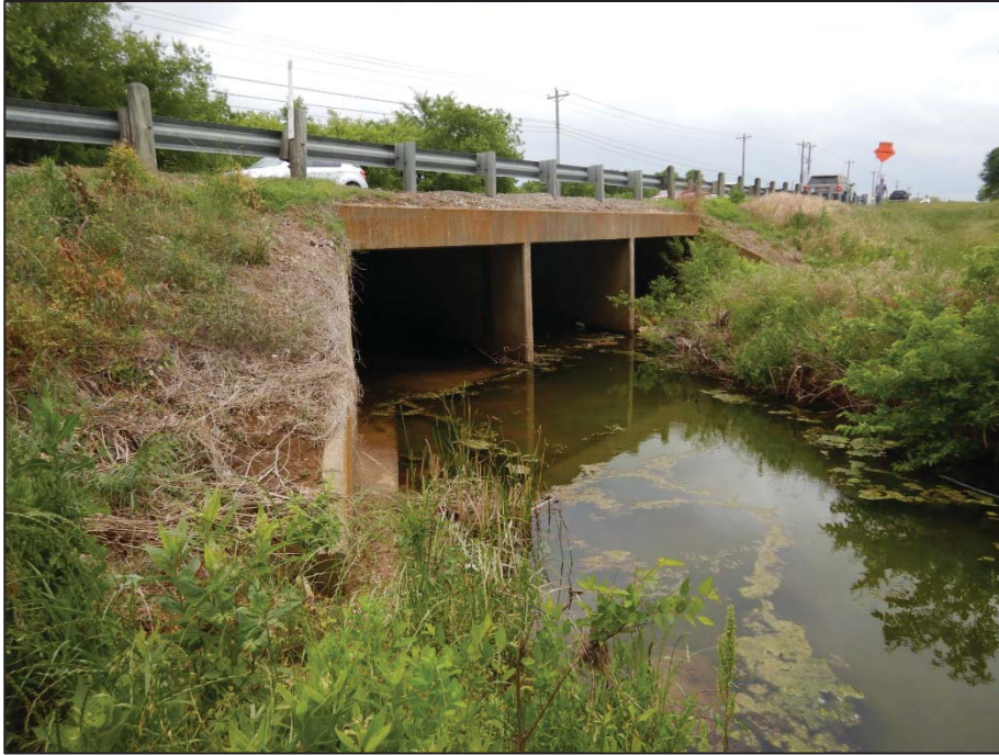
Photo 93: View looking southeast toward Crossing 14 – tributary to Pecan Creek (US 377 southbound side).
