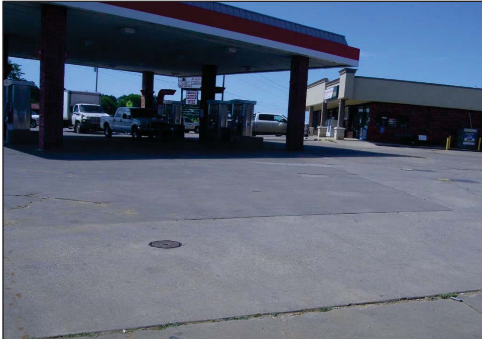
Photo 43: View looking south towards a monitoring well at the Chaparral Plaza LPST and PST site at 704 S. US 377, Aubrey, TX 76227 (HazMat Site 28). The tank hold is at the right of the photo. Date of Photo: 5/6/20.
