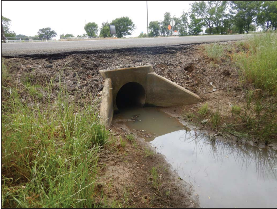
Photo 97: View looking west toward Crossing 15 – tributary to Cantrell Slough (US 377 northbound side).
