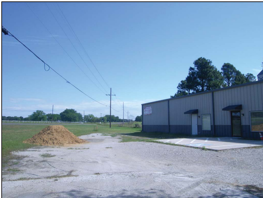
Photo 22: View looking northeast from Black Jack Rd toward ATX Auction House, a potential displacement (Disp 4) at 556 E Blackjack Rd, Pilot Point, TX 76258. Date of Photo: 5/6/20
